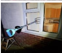
A picture of a property where a pitch fork used from the garden to prise open a window
